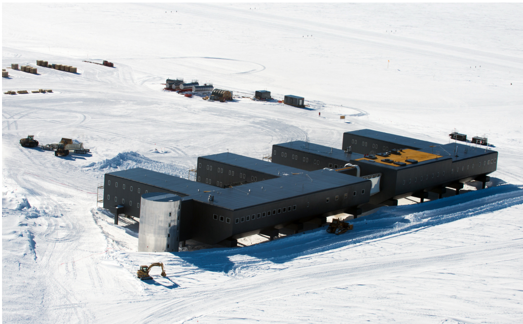
Figure 44: Aerial view of the Amundsen-Scott South Pole Station.
